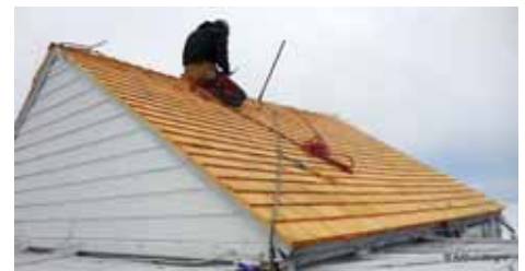
Dustin - Finishing the ridgecap (above), Standing by the finished product (below)
