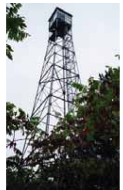
Many of Wisconsin's towers have enclosed ladders rather than stairs.
