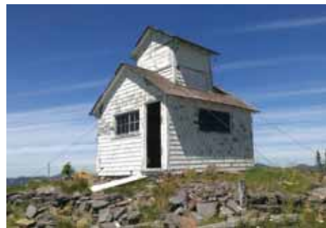
Priscilla Peak Lookout in 2013. Taken off the cabin rental program due to lack of use, Priscilla is beginning to show the need for some TLC. Luke Channer photo
